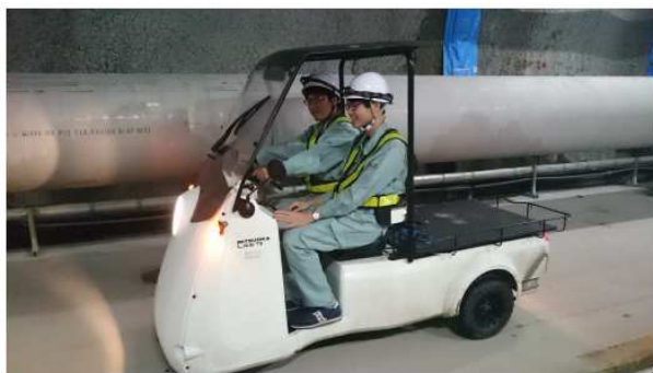
FIG. 10. Each worker is equipped with a helmet, working cloth, reflective vest and headlight for work inside the tunnel. Small electric carts are used for the 3-km transport from the central area to the end station.
