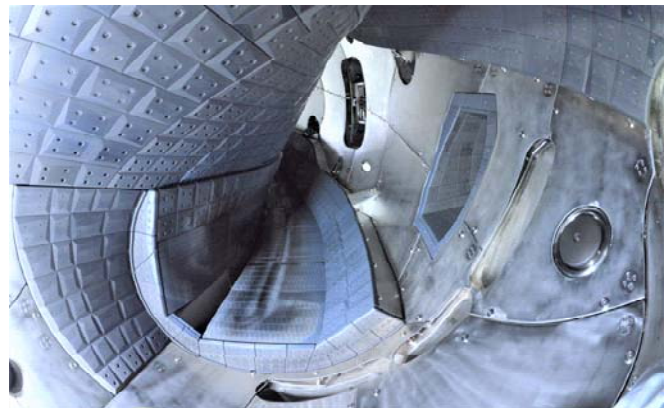
Fig. 1. View into the W7-X plasma vessel just before the start of OP 1.2b. Shown here is module 2 with a glow discharge electrode on the right wall, an NBI entrance port (shielded by C-tiles) and one of the bottom TDU. This consists (from the right) toroidal divertor closure, outer baffle, horizontal target plate, divertor pump slit, horizontal target plate and inner baffle. On the front, the vertical divertor closure is visible. On both of the target plate, the traces of the separatrix are well visible. (courtesy G.Wurden/LANL)
